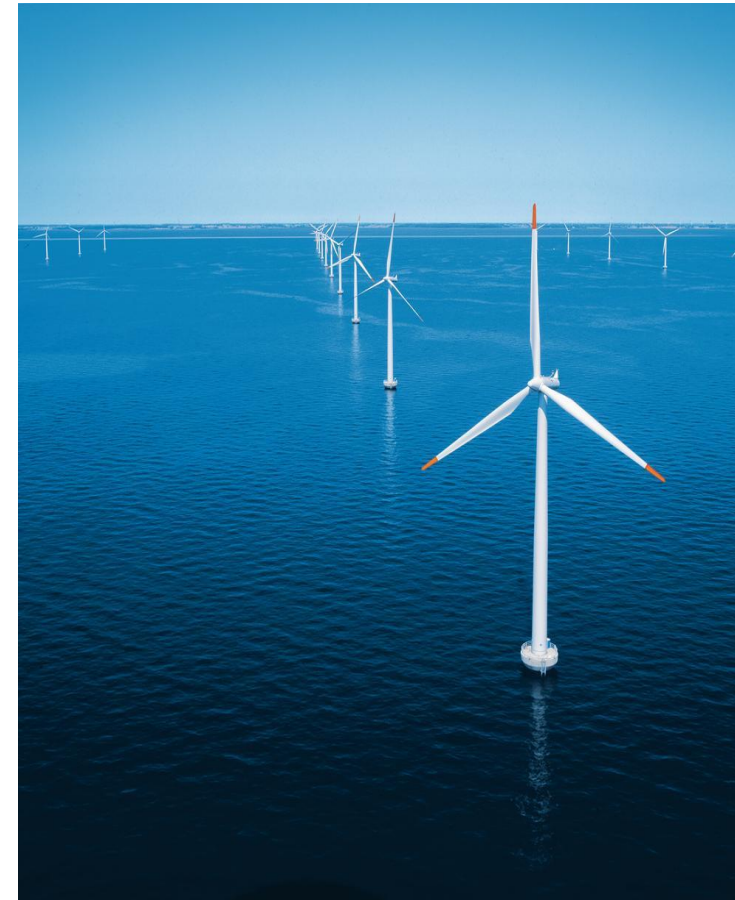
Nysted Offshore Wind Farm, 72 units 2.3 MW, 165.6 MW, SWT-2.3-82
