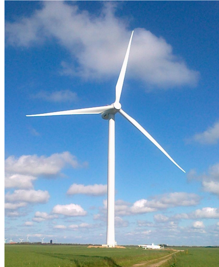
Prototype installation Høvsøre, Denmark
