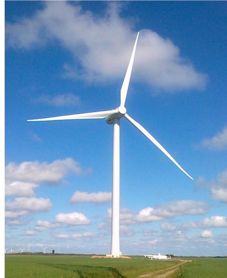
Prototype installation Høvsøre, Denmark
